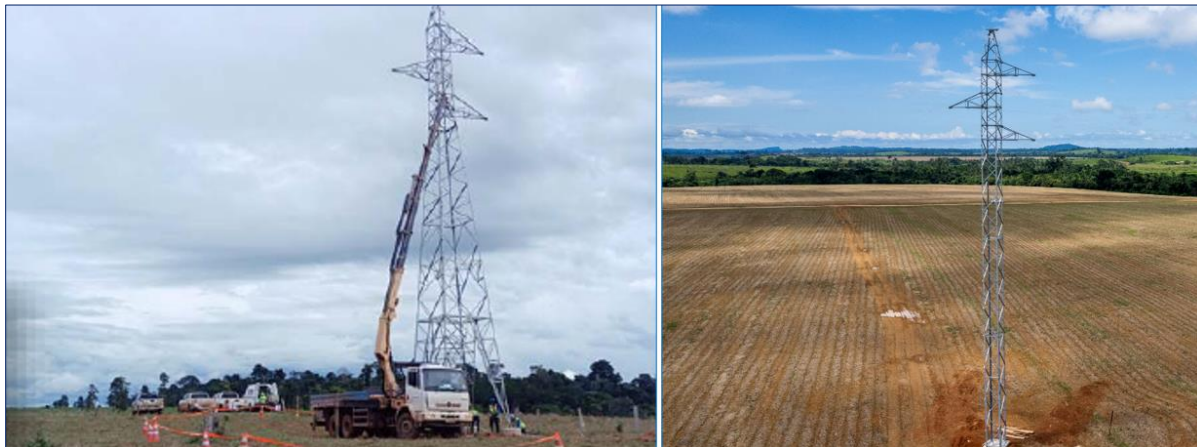
Figure 4: Transmission line erection
