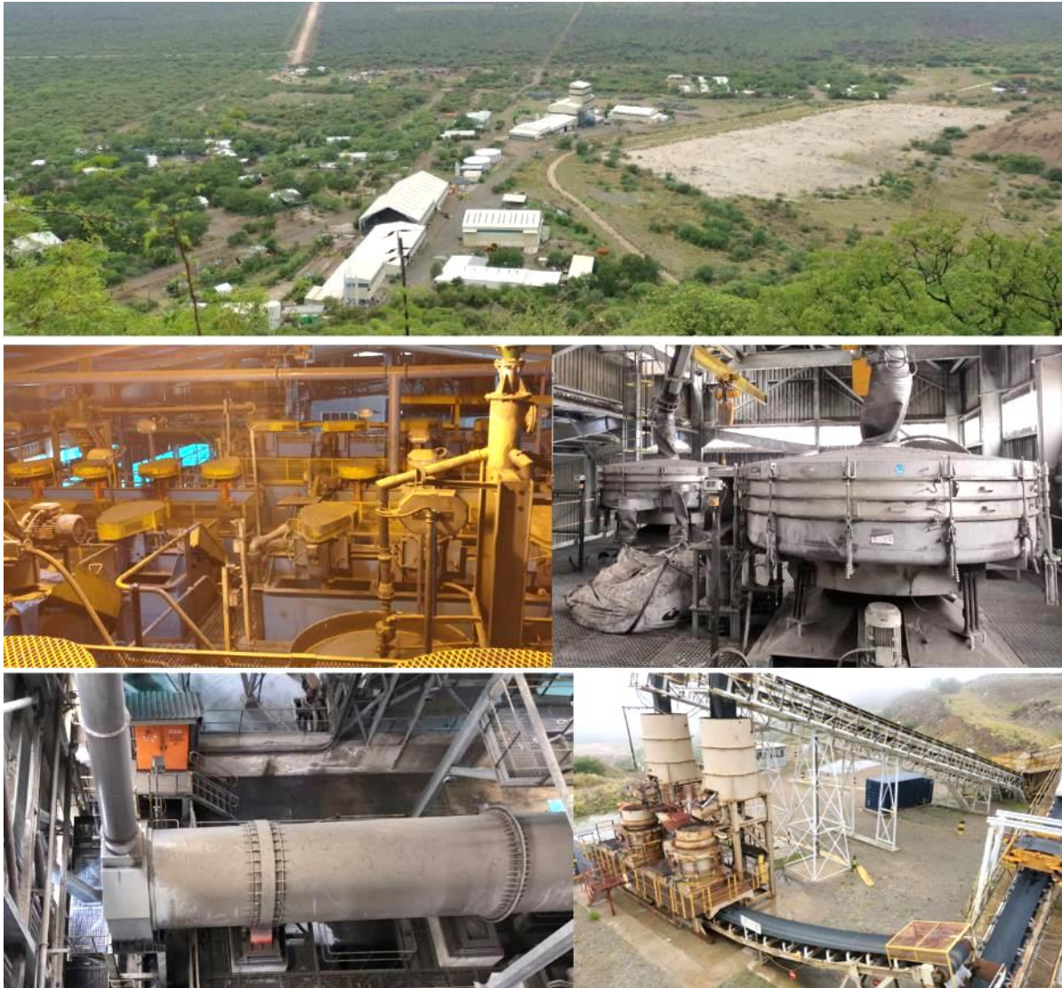
Figure 6 (A) Plant layout, (B/C/D) plant internal aspects and belts and conveyors
