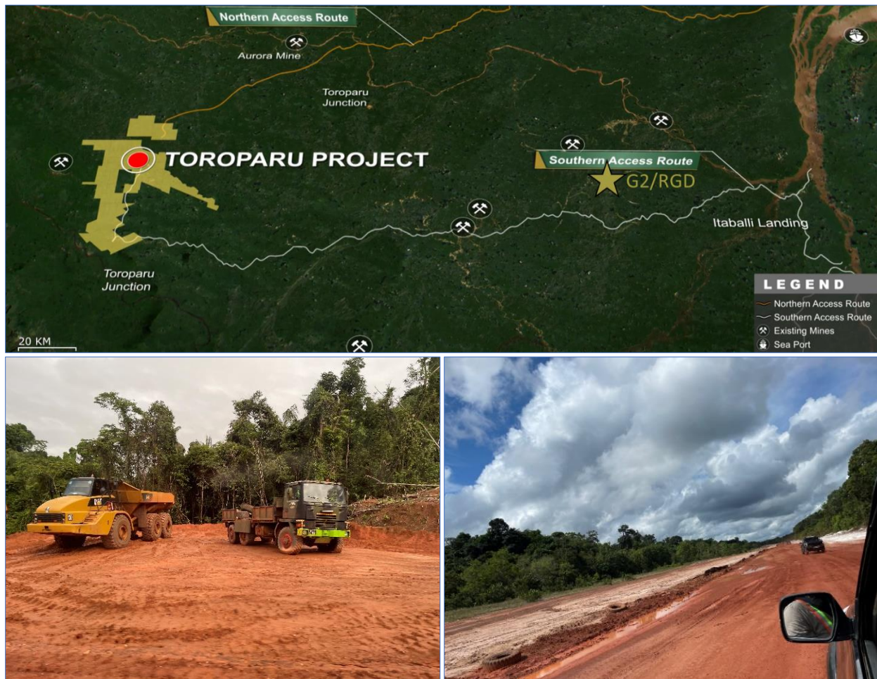
Figure 5. (A) regional plan map showing southern access route to Toroparu with approximate G2/RGD location (B) active construction equipment, and (C) upgraded southern access route
