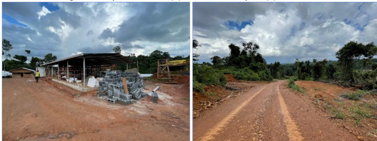
Figure 5. Camp infrastructure (A) new stores facility and (B) access road
