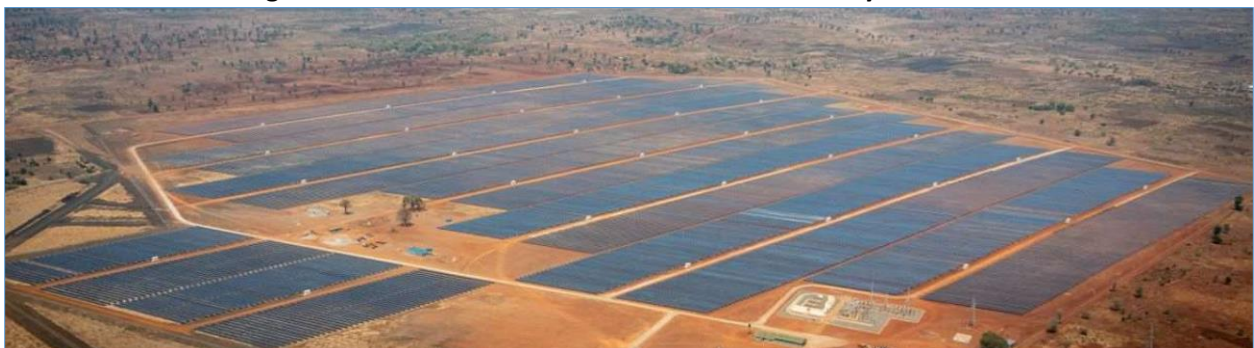
Figure 4. A 60Mw solar farm commissioned recently in Malawi
