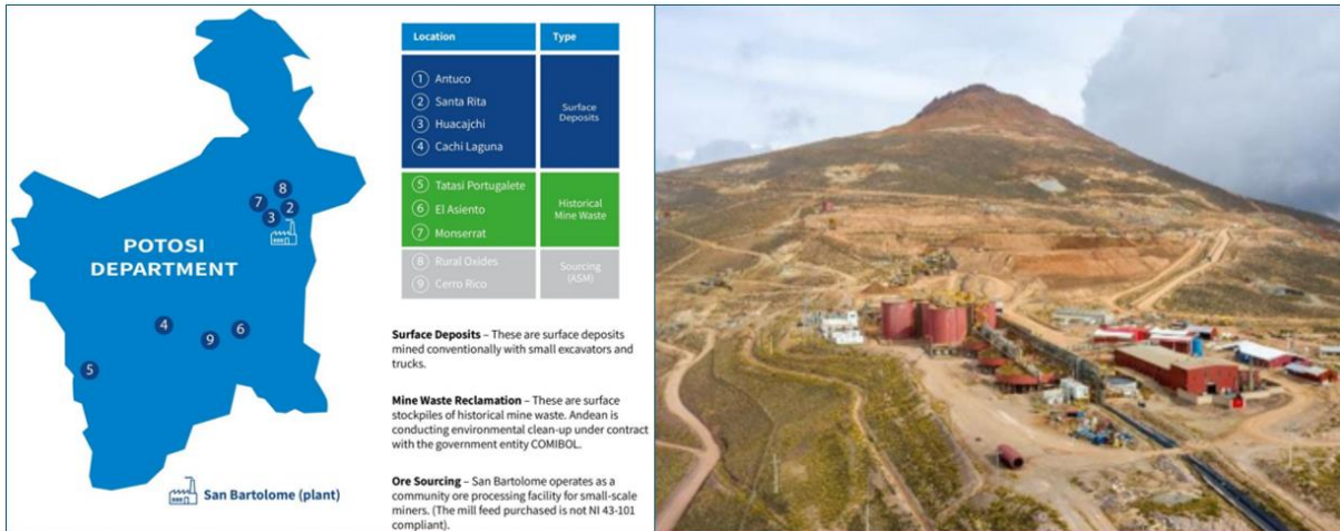
Figure 11: (A) Map of asset locations within Potosi Department; (B) San Bartolome processing plant
